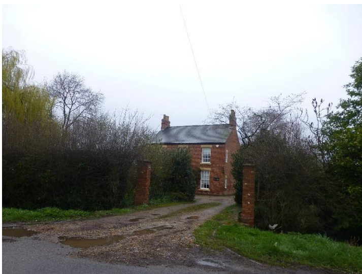
Plate 45: View of Meaburns, looking east
