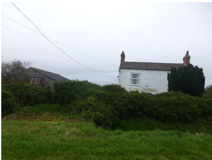
Plate 44: View of Moor Farm, looking east
