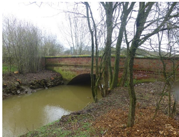
Plate 13: View of bridge adjacent to Dirtness Cottage
